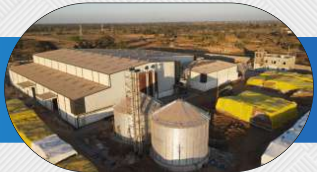
Project – Maa Food Products, Raipur Chhattisgarh 63000 Sq Feet Project Type – Rice Mill Shed
